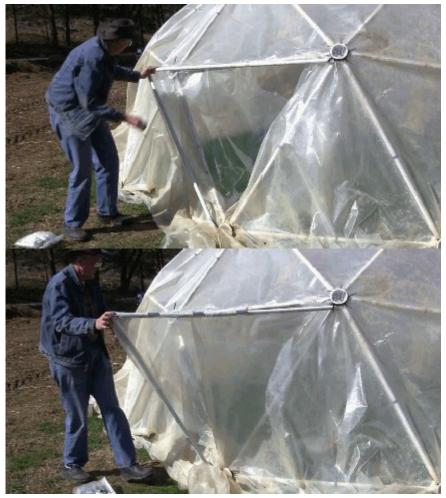
Patch any holes with clear tape. You can attach a clear plastic flap on the outside over the top of the opening to hold the door closed and to help insulate the dome.
