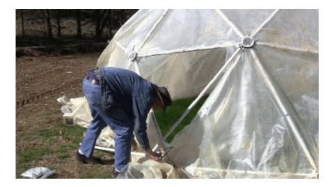
To make the door, connect the loose ends of the two struts together using two zip ties.
