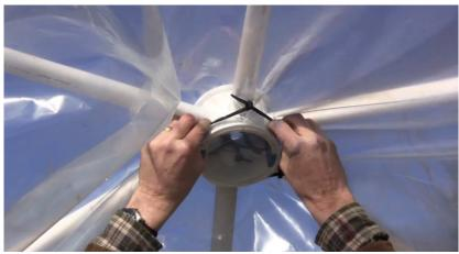
Pull the covering to the next hub, and take up any slack in the covering between the hubs. Secure the covering to all of the hubs in the interior of the dome.
