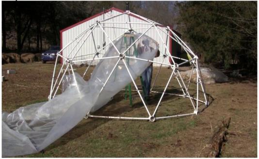
Get under the covering and place the marked center of the covering over the hub at the top of the dome. Have 3 zip ties in a daisy chain ready to cinch down the covering over the hub. You may need one or more people to help you do this.
