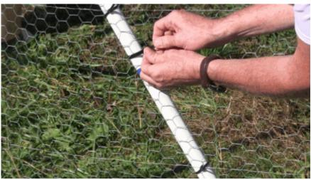
Loosely attach a Zip Tie just above the blue or red tape on the strut.
