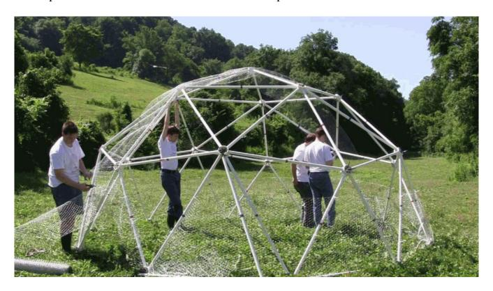
Cover the remaining openings with large sections of chicken wire.
