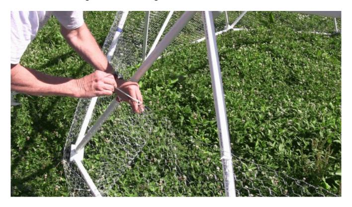
To tighten the chicken wire, overlap it and secure by threading a zip tie through the overlapped layers of mesh, and then tighten the zip tie.
