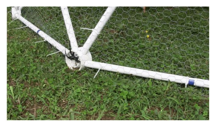
Use at least 4 Zip Ties on each strut to secure the wire to the struts.
