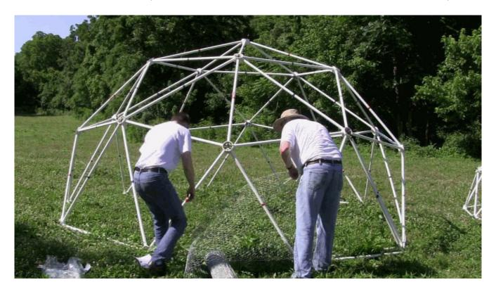
Unroll some of the chicken wire, and attach the wire to the struts along the edge of the door opening using the smaller 50 lb zip ties.
