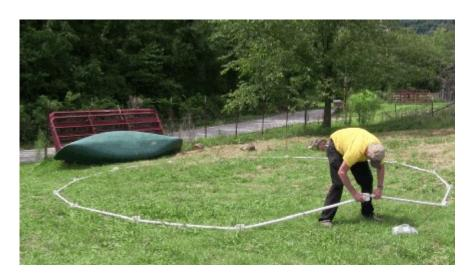
Before connecting, make sure each Hub is pointing upwards, with one of the large openings laid flat on the ground, and with the smaller openings for the struts in a horizontal position.
