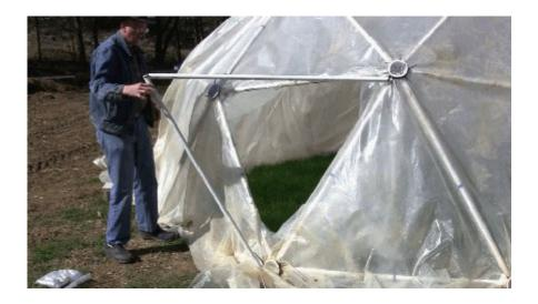
Pull the loose plastic flaps up to the door, and attach the plastic to the door with clear tape or greenhouse clips.
