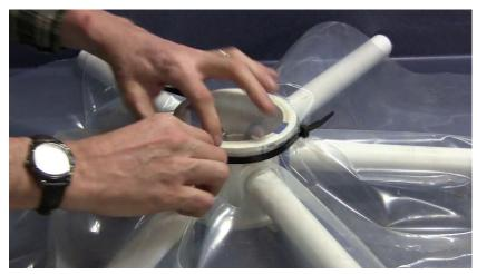
It is easier to attach two layers to the dome if you start with the covering on the inside of the dome. To do this, you will need to find the exact center of your covering material, so that it can be attached to the center, or top, of the inside of the dome.
