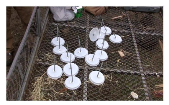
The Test Caps and carriage bolts will be used on the hubs at the top of the first tier of the dome. Fold any excess greenhouse covering over the hubs on the top of the first tier to make a pleat. Insert the carriage bolt through the pleat, and through the center ring of the hub.
