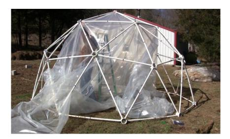
Pull the outside covering over the outside of the dome. Use Zip Ties to secure the outside covering to the hubs on the sides and on the bottom of the dome.
