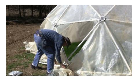
To make the door, connect the loose ends of the two struts together using two zip ties.
