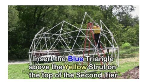
Step 18. Connect the Top of the 3rd Tier with 10 Blue Struts.
