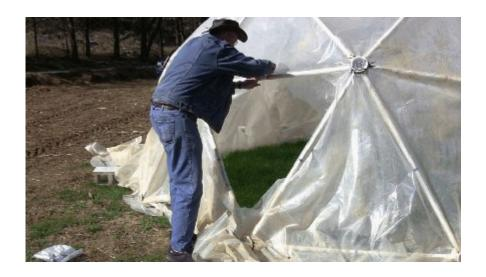
Tie a Heavy Duty Zip tie through the end of one of the Blue Struts, leaving a large loop in the Zip Tie.
