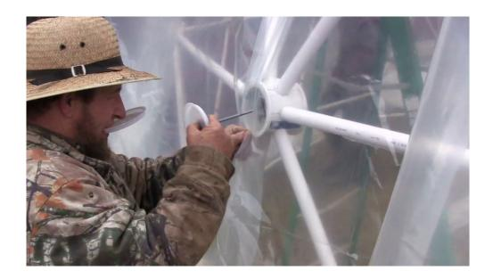
Push the Test Cap into the hub opening, securing the greenhouse covering to the hub. On the inside of the dome, thread a Test Cap over the carriage bolt, and secure with a washer and nut.
