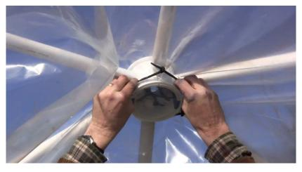
Pull the covering to the next hub, and take up any slack in the covering between the hubs. Secure the covering to all of the hubs in the interior of the dome.
