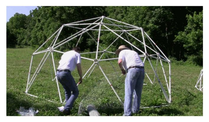
Unroll some of the chicken wire, and attach the wire to the struts along the edge of the door opening using the smaller 50 lb zip ties.
