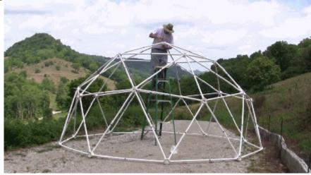
Secure the Struts with Zip Ties. The Dome is Complete!
