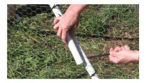
Let the handle hang down so that you can see where the bottom of the handle meets the strut. Then loosely attach a Zip Tie around the strut near the bottom of the handle.
