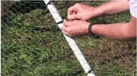
Loosely attach a Zip Tie just above the blue or red tape on the strut.
