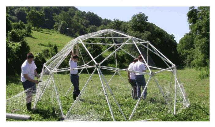
Cover the remaining openings with large sections of chicken wire.
