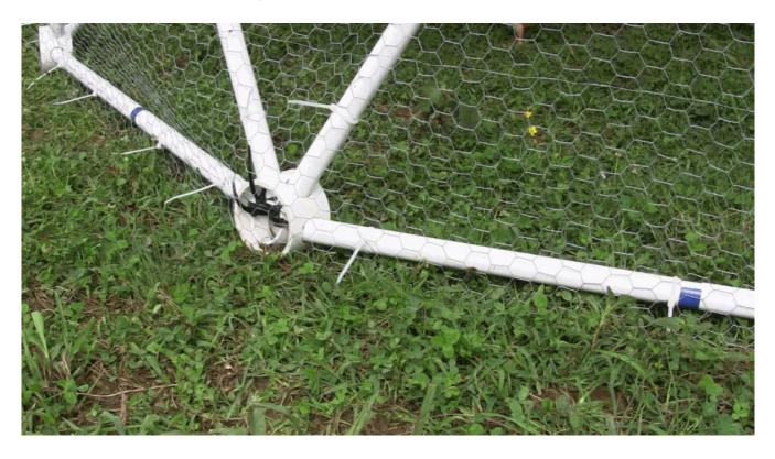
Use at least 4 Zip Ties on each strut to secure the wire to the struts.
