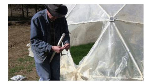
Daisy chain 3 zip ties together as shown in "How to Attach a Greenhouse Cover", and loop them through the zip tie on the end of the strut.
