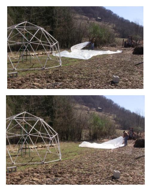
Find where the double fold is, and make a large, visible mark with an ink marker to mark the center of the covering.
