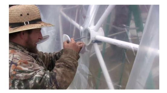
Push the Test Cap into the hub opening, securing the greenhouse covering to the hub.
