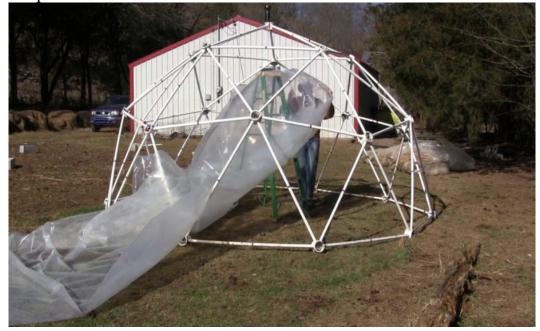
Get under the covering and place the marked center of the covering over the hub at the top of the dome. Have 3 zip ties in a daisy chain ready to cinch down the covering over the hub. You may need one or more people to help you do this. Lift the covering up over the hub, and secure it to the center top hub with zip ties.
