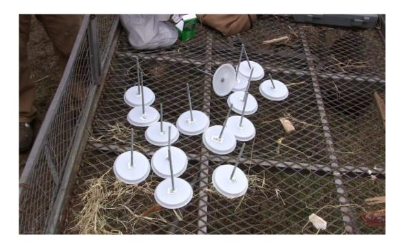
The Test Caps and carriage bolts will be used on the hubs at the top of the first tier of the dome. Fold any excess greenhouse covering over the hubs on the top of the first tier to make a pleat. Insert the carriage bolt through the pleat, and through the center ring of the hub.
