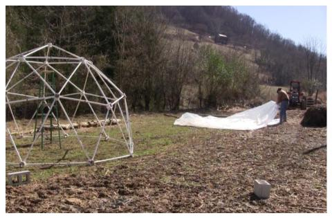
Find where the double fold is, and make a large, visible mark with an ink marker to mark the center of the covering.
