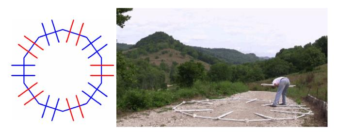
Spread each of the two struts to make a triangle.
