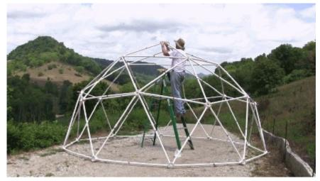
This will be a <u>tight fit</u> as the last pieces will lock the dome together. You may have to stand near the top of the ladder to apply force.
