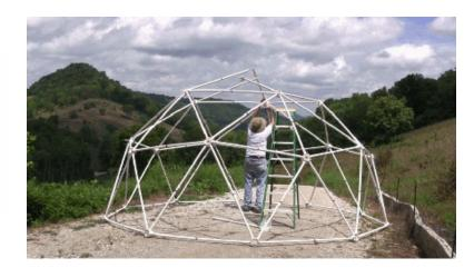
Using a stepladder, move the Top Red Hub up and down to insert the Struts into the Hub.
