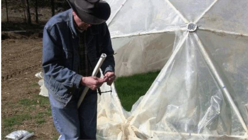
Daisy chain 3 zip ties together as shown in “How to Attach a Greenhouse Cover”, and loop them through the zip tie on the end of the strut.
