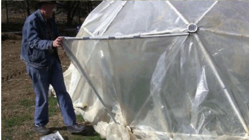
Patch any holes with clear tape. You can attach a clear plastic flap on the outside over the top of the opening to hold the door closed and to help insulate the dome.
