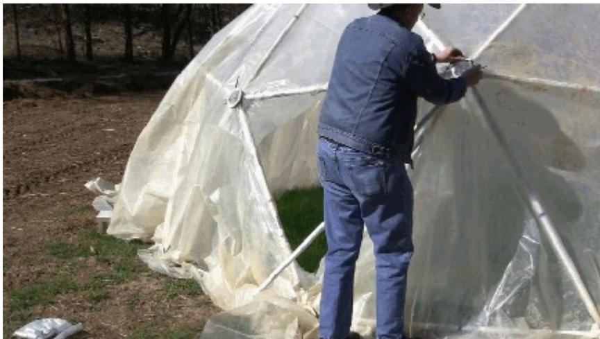
Take the second strut, and attach it in the same way to the hub at the bottom of the opening.
