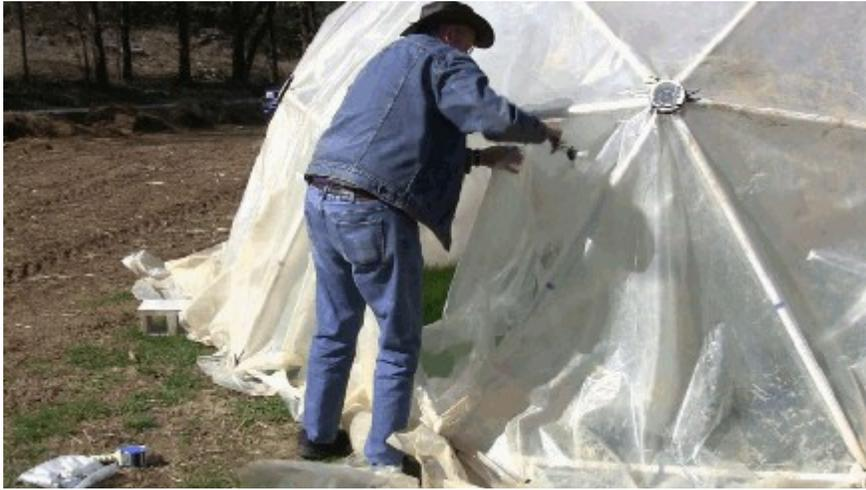
Tape the loose plastic along the two cut sides to the struts, leaving the flaps to be used for the door.
