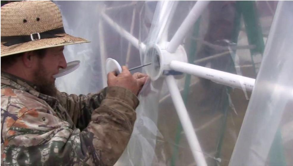
Push the Test Cap into the hub opening, securing the greenhouse covering to the hub.
